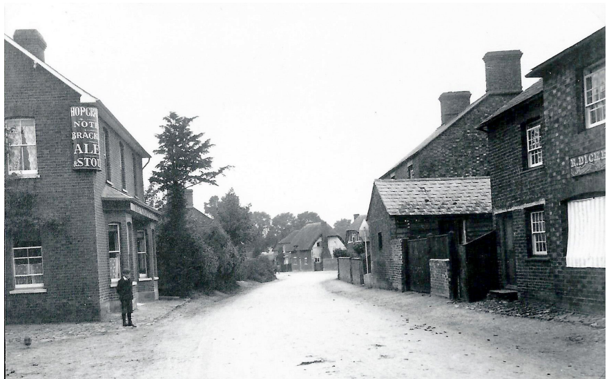
Church Villas, the terrace with the large gable end chimneys on the right, was the site of John Faulkner's dung-cart business. The Kings Head pub on the left was the source of his casual labour.
