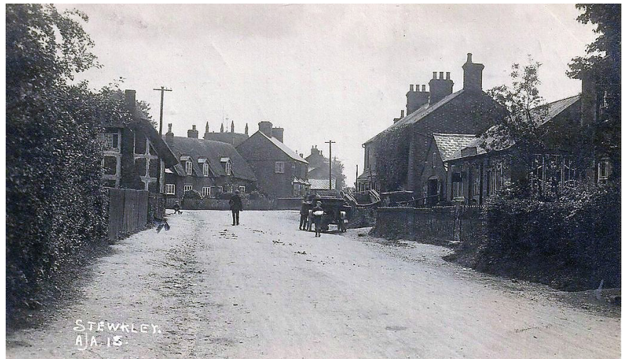
The site of the Dickens Brothers' wheelwright workshop at 27 High Street North
