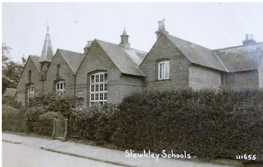
Stewkley School, High Street North, 1930s
